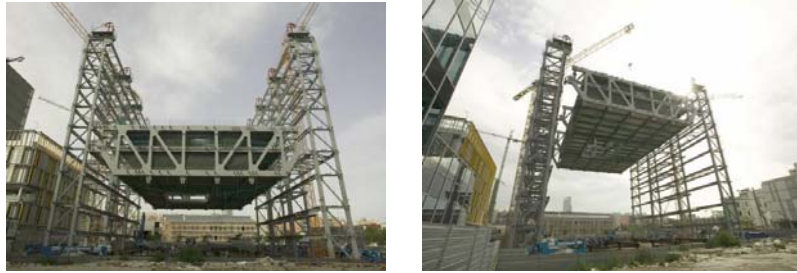
Images of the structure being hoisted into position
