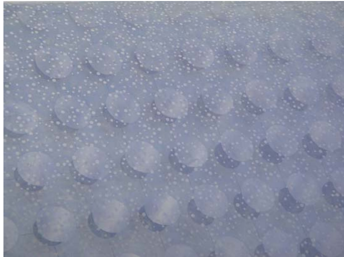
Seen up close, the ETFE serigraphy presents diverse layers of solar exposure
