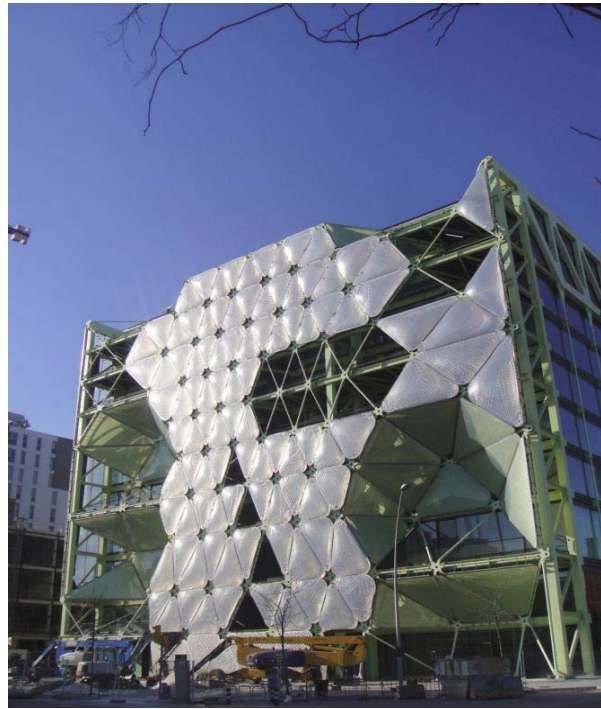
Media-TIC at the intersection of Sancho de Ávila and Roc Boronat
