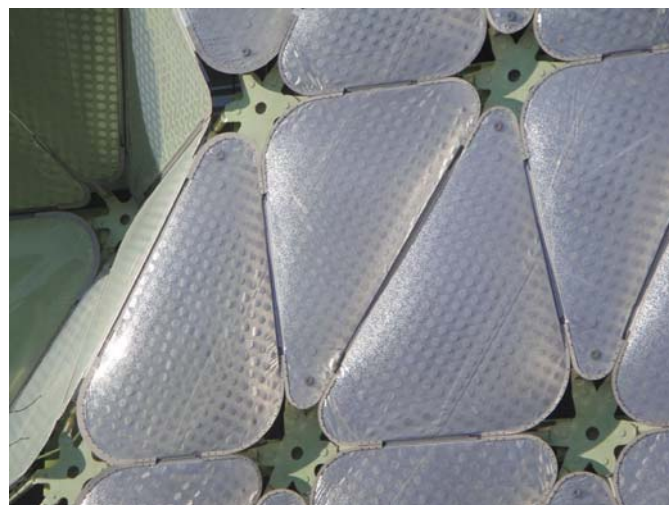
Detail of one of the mobile bags that function as a solar screen
