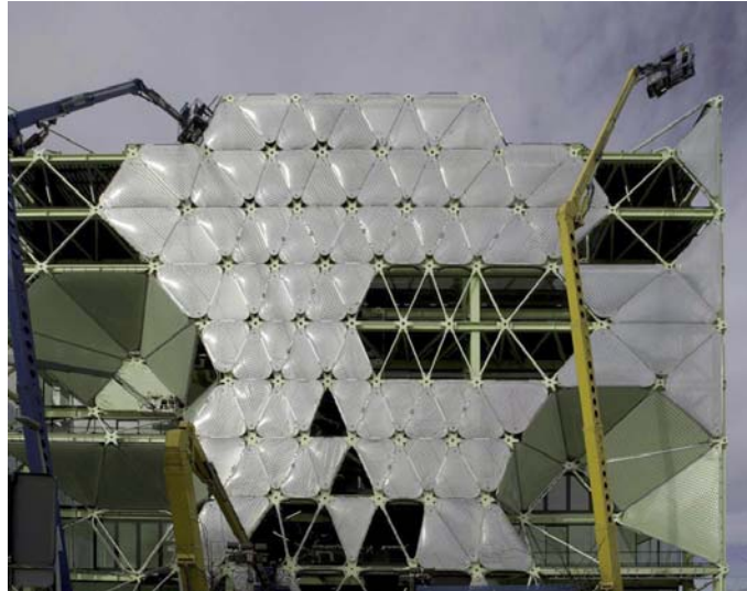
Works involved in covering the façade, with the characteristic ETFE skin
